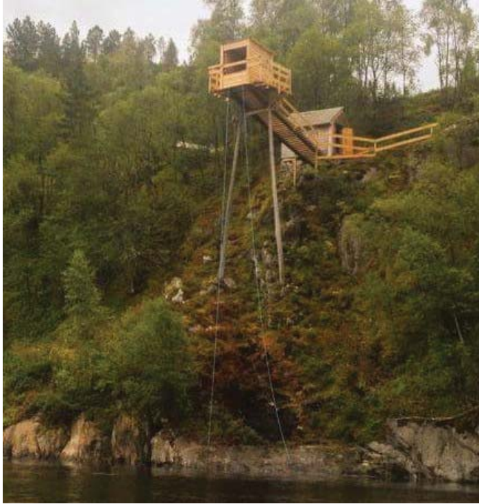
Photo 10.4: A recently renovated salmon trap at Askildneset. This was a well-developed fishing technique whereby a seine net - a bag that is open at one end – is set in the sea immediately beneath the trap. The salmon fishermen sit at the top of the trap, high above the fjord, and keep a sharp eye on the water. When a salmon enters the net, they close it by drawing a line. Photo: Erling Kleiveland.
